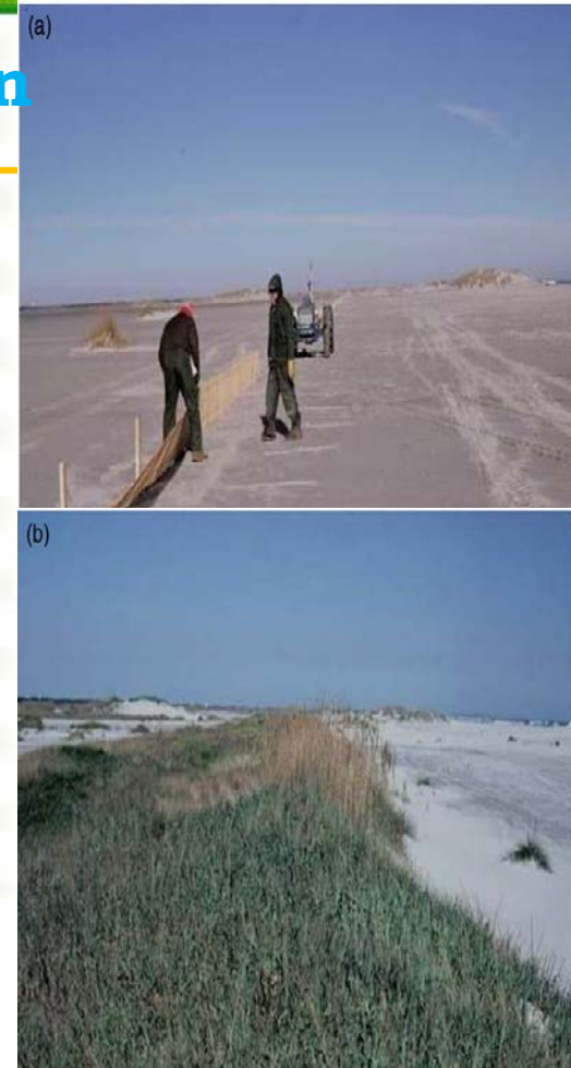
Figure 2 (a) Installation of a sand fence for dune restoration in January 1978. (b) The same site in October 1981.
